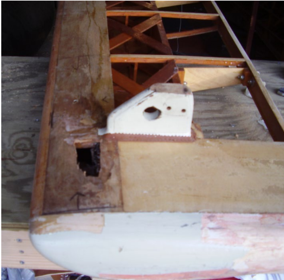
Rotten wood replaced on the bottom of the right wing.
